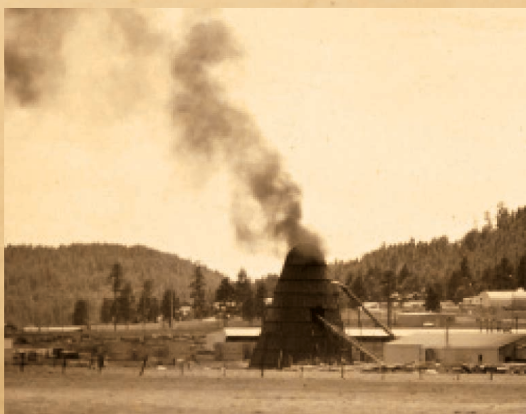
A-frame burner, formerly used to destroy waste bark
