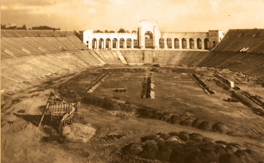
Early Coliseum construction — Photo Courtesy of the LA Memorial Coliseum Museum
